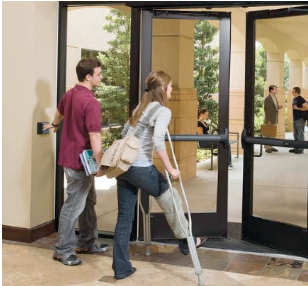
Entrance door with automatic or push button opening system requiring little or no effort from the user
